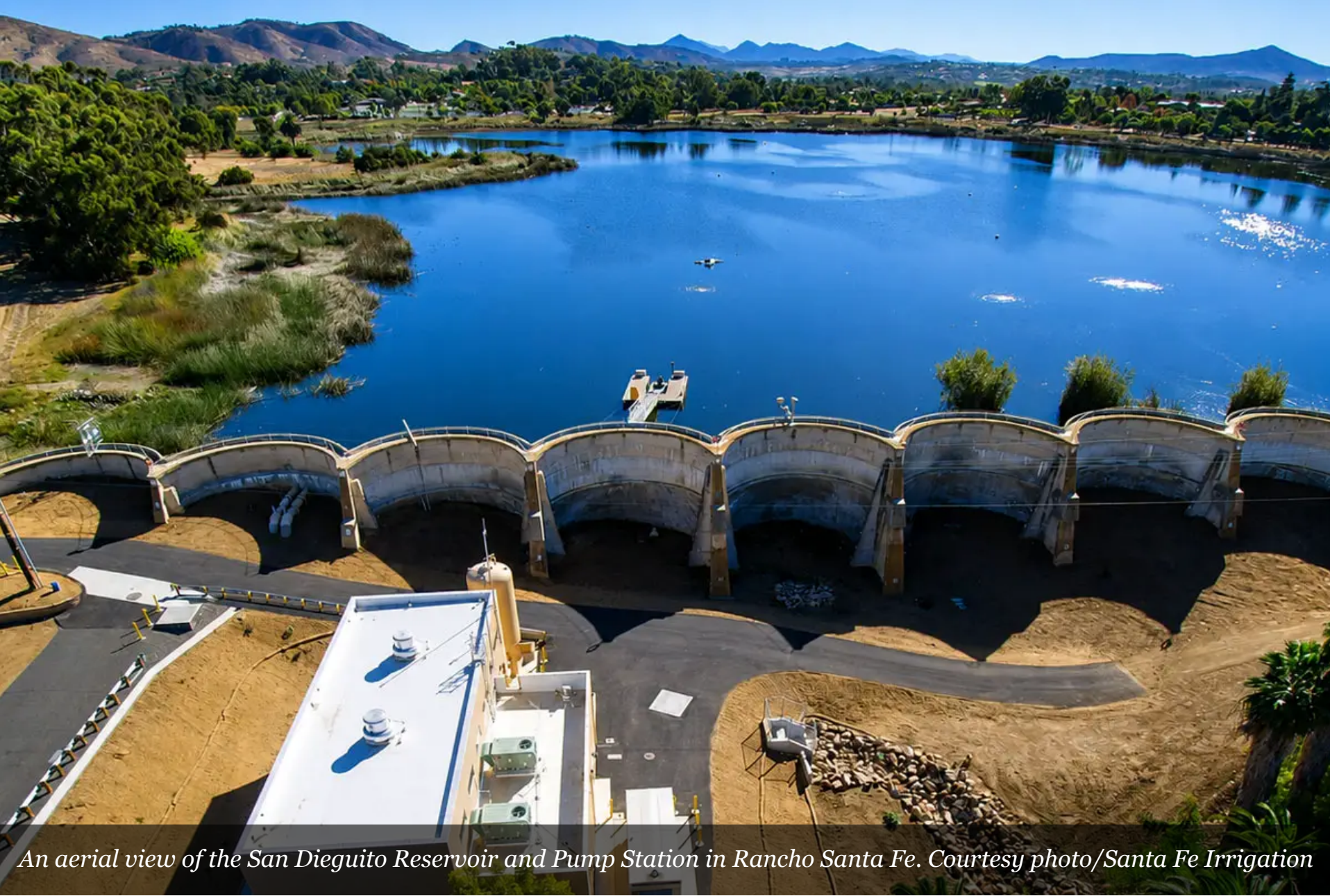
An aerial view of the San Dieguito Reservoir and Pump Station in Rancho Santa Fe. Courtesy photo/Santa Fe Irrigation
