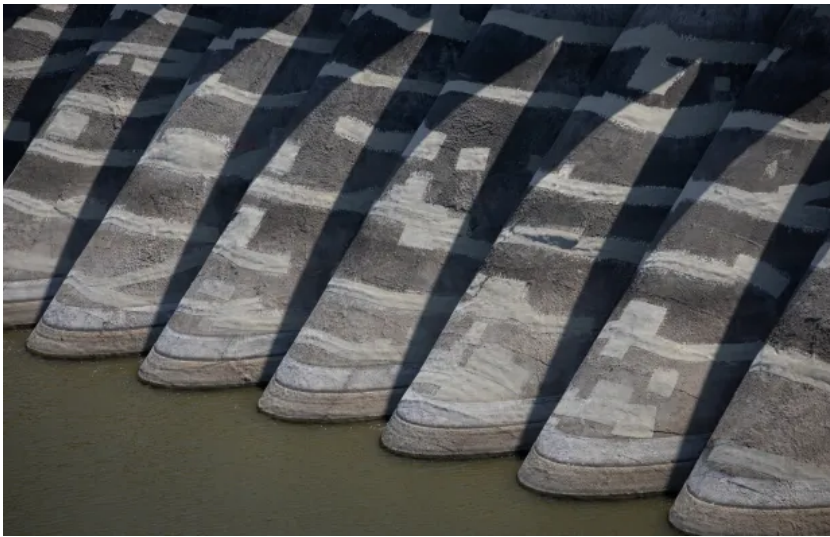
Lake Hodges Dam on Wednesday, Aug. 13, 2025 in San Diego. (Ana Ramirez / The San Diego Union-Tribune)
