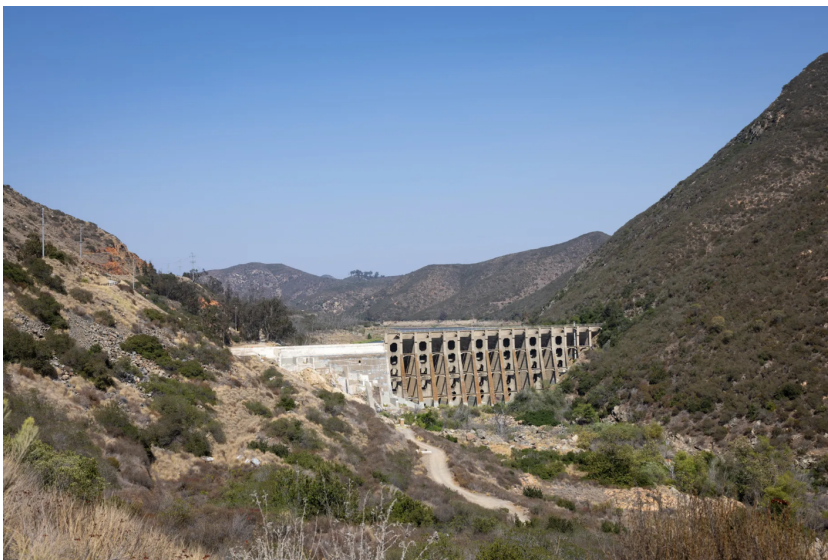
Lake Hodges Dam on Wednesday, Aug. 13, 2025 in San Diego. (Ana Ramirez / The San Diego Union-Tribune)
